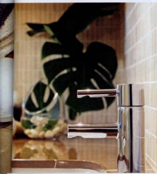
The spout had to be custom made to clear the edge of the bath.
